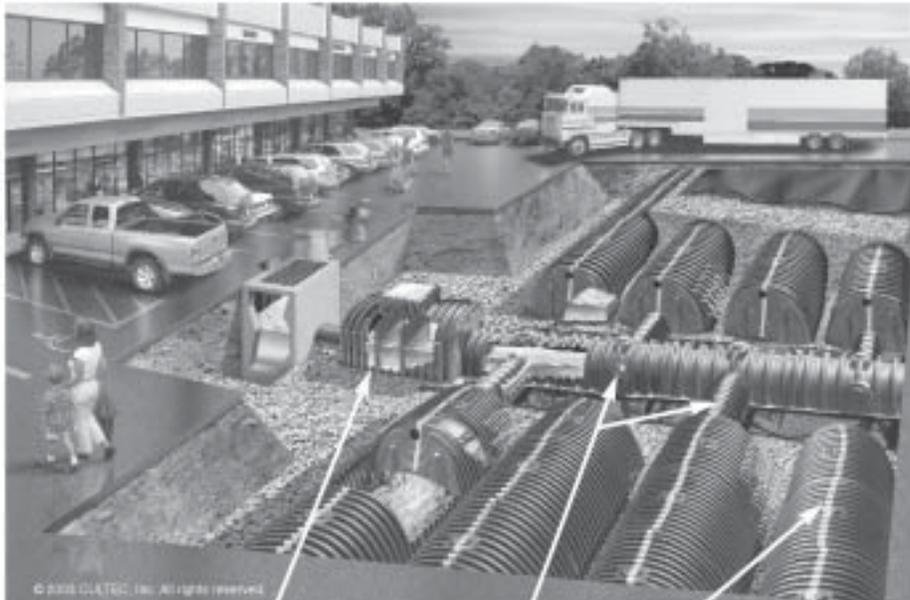
CULTEC plastic chambers for underground stormwater detention/retention eliminate the liability associated with surface ponds. The chambers are lightweight and easy to maneuver around a job site, so heavy equipment use is kept to a minimum, resulting in less land disturbance. The open bottom and perforated sidewalls provide higher infiltration capability and groundwater recharge.
